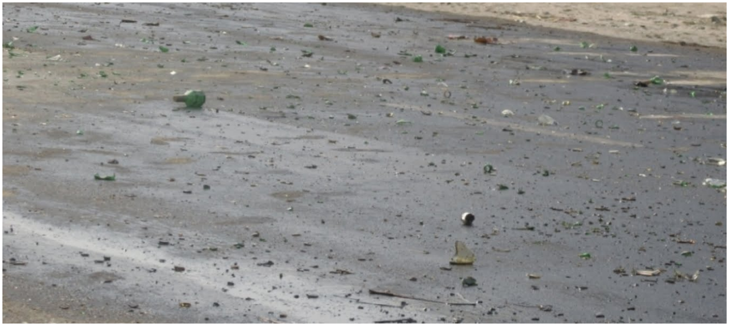
Broken glass covers the road. Image: Bhola Paswan
