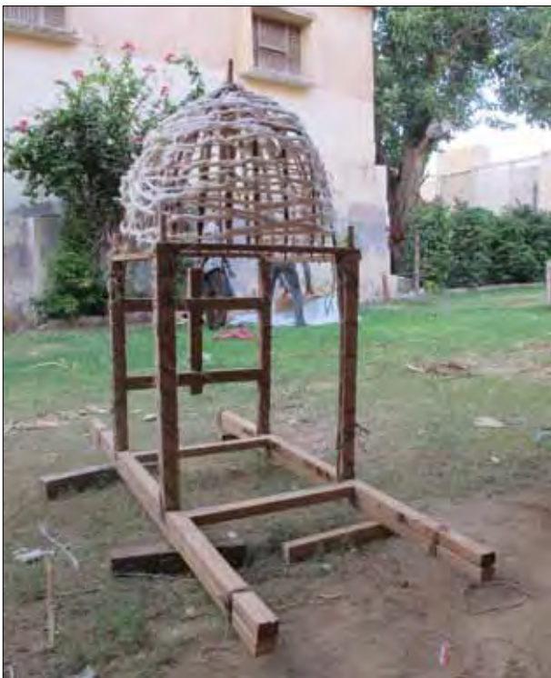
Fig. 6 The baikuṅṭhī for Smt. Bacchāvāt under construction, Sardārśahar 5.10.2014 (Photo: Peter Flügel)
